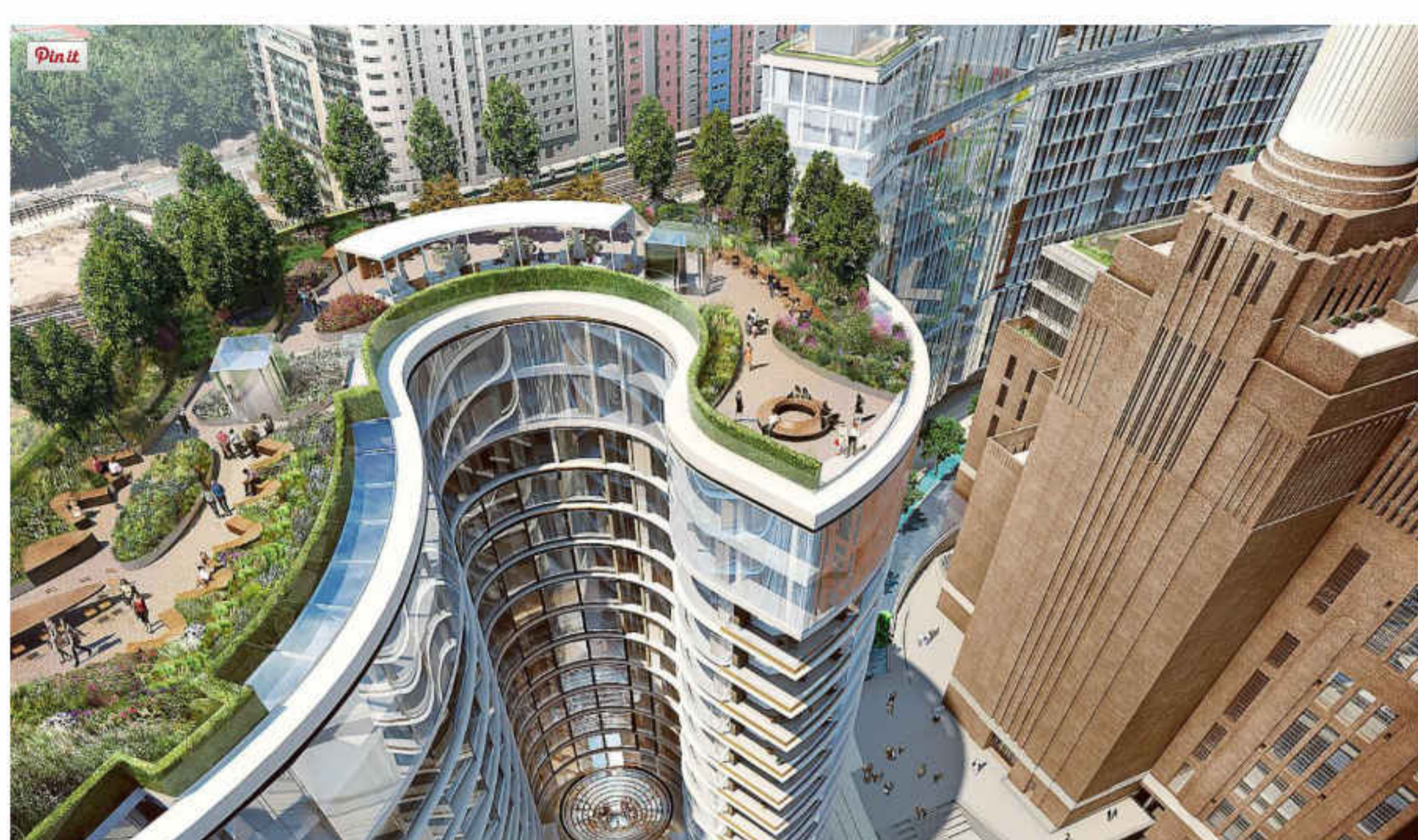
High point: the rooftop gardens at Battersea Power Station — residents can also flex their green fingers on the scheme's allotments
